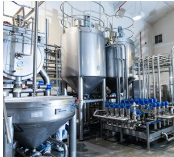
► Dairygold Food Ingredients UK Cultured Dairy site in Leeds.
