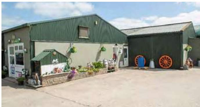
The Herlihy farm yard.
